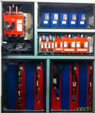
Typical five VFD module configuration (shown inside cabinet and with doors closed)
