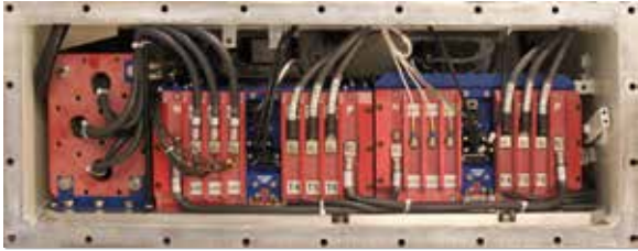
14CM Continuous Miner installation
