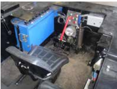
Q800 drive installation (also shown with digital display and operator station)
