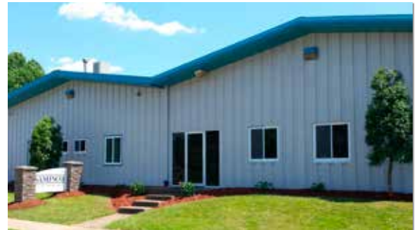
Our Huntington, WV facility includes our panel shop, rebuild /repair workshop, and motor warehouse.
