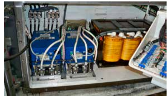
Two drive system for continuous miners
