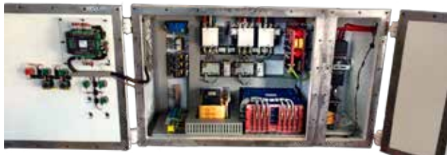
Feeder Breaker Controller Installation
